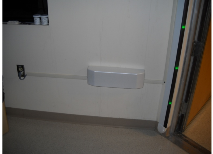
Power Supply wall bracket can be configured vertically or horizontally to cover electrical outlet for clean install
