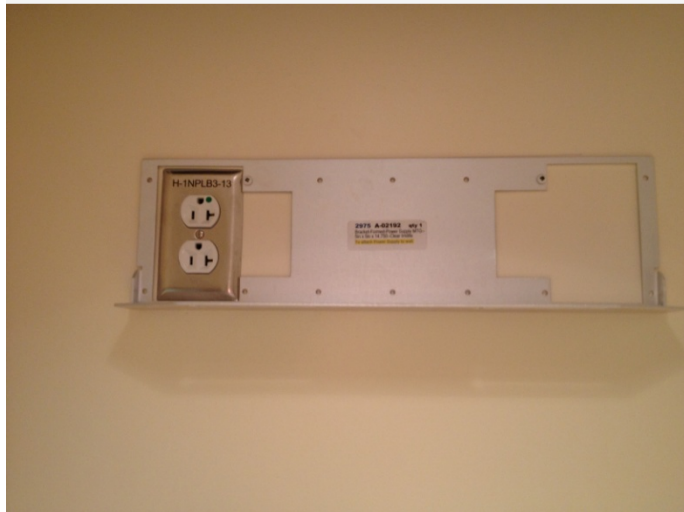
Power Supply of typical IN MAGNET room installation finished outlet covered
