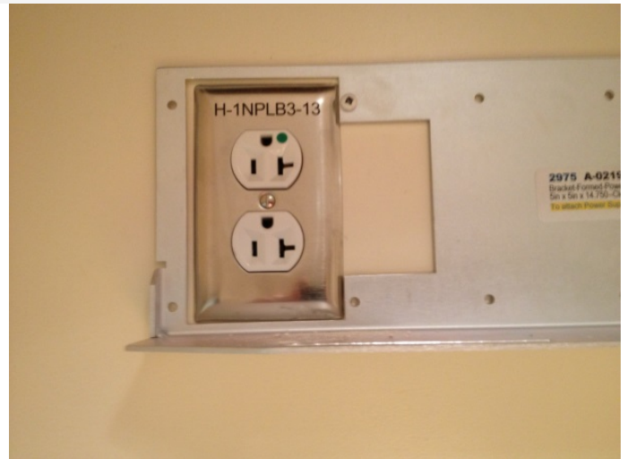
Power Supply of typical IN MAGNET room installation finished outlet covered
