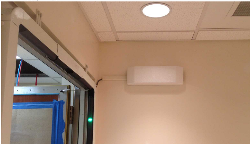
Power Supply of typical IN MAGNET room installation finished outlet covered
