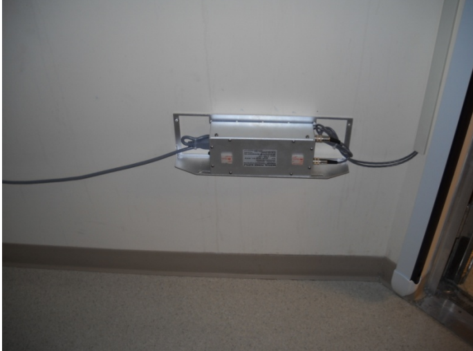
Power Supply wall bracket can be configured vertically or horizontally to cover electrical outlet for clean install
